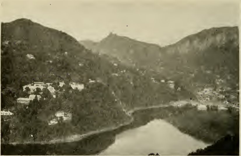
Wellesley High School (at left) on the mountainside, overlooking shining Naini Tal
